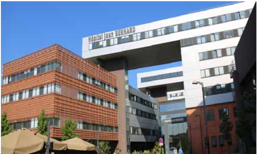
Figure 4. Bioclimatic facade system in Jean Bernard Hospital, Groupe 6, France, 2010
