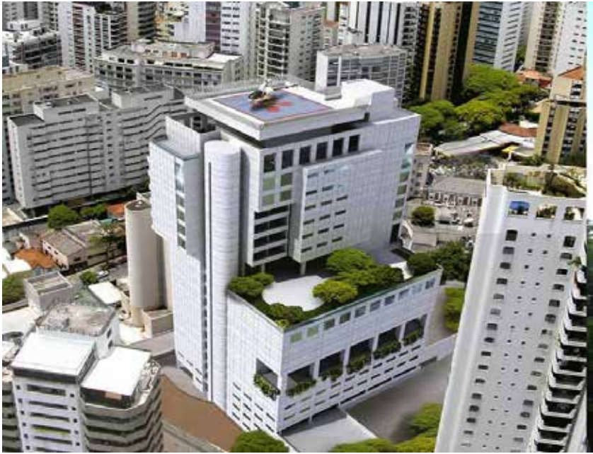
Figure 5. Bioclimatic facade system in Samarito Hospital, Brazil, 2009
