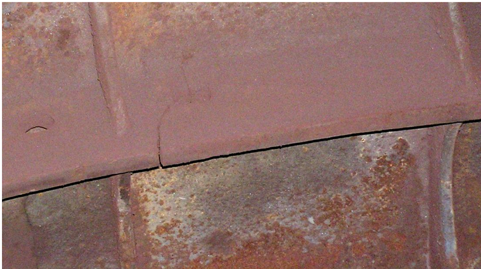
Figure 1. Fracture in the annular side of the adjacent tubing
