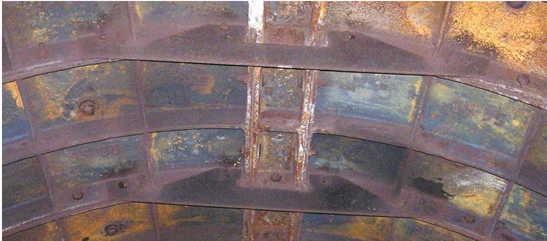
Figure 4. Metal plates in the vault of the tunnel
