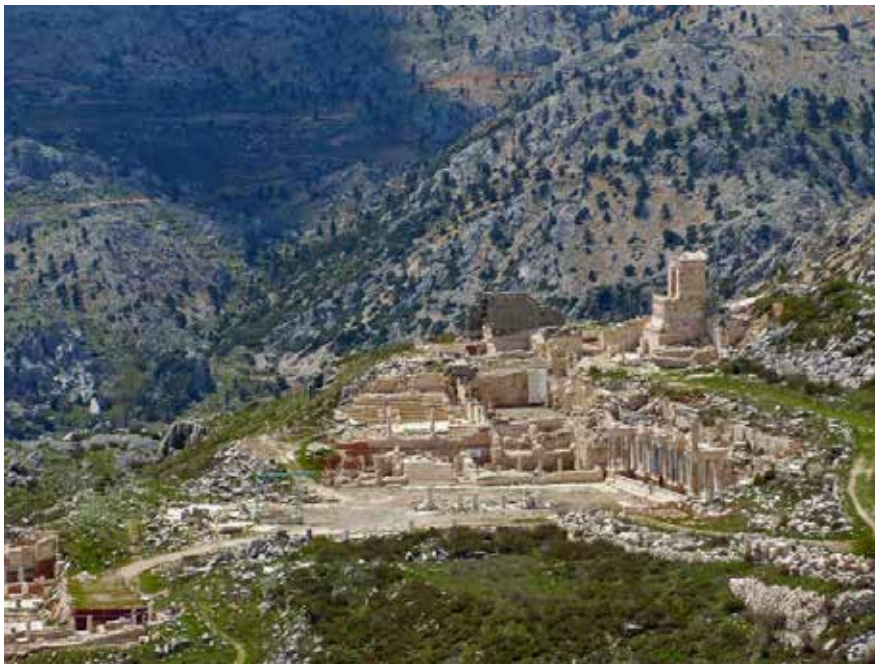
Fig. 13. General view of the upper agora of Sagalassos. Current state (Panchenko S., Soboliev V. 2014)
