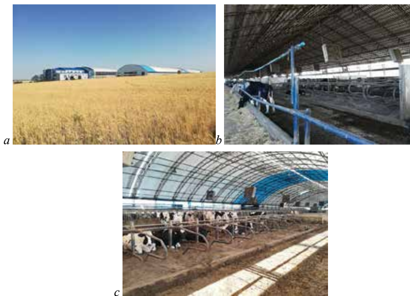
Figure 1. Monoblock of the dairy complex with uninsulated rooms of different types ( a – the appearance of the dairy complex; b – cowshed carcass type; c – cowshed hangar type)
