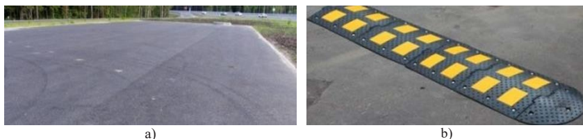
Figure 2. Areas of the road surface for the experiment: a) – asphalt road; b) – asphalt road with an obstacle
