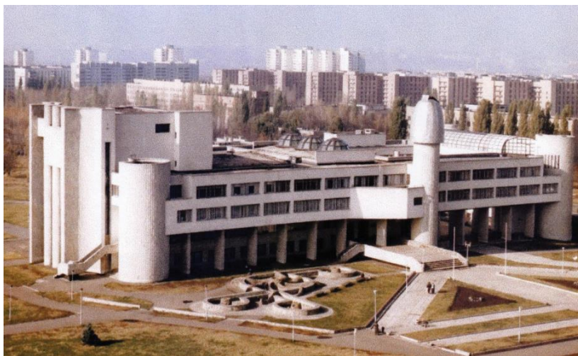
Fig. 1. General view of the building of CI KhPCYC
