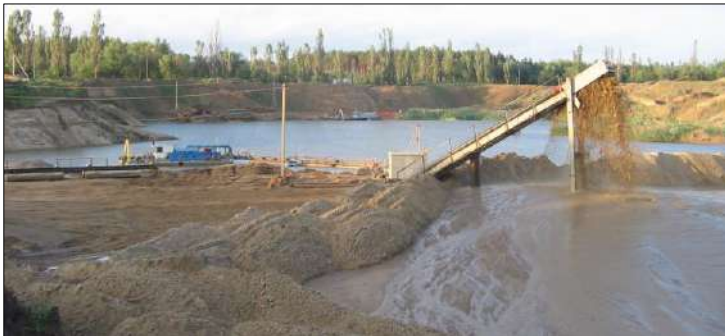
Fig. 3. Use of an inclined screen for sand separation
