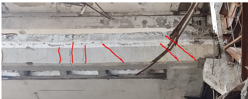
Figure 2.7 – Cracks in the crossbar at the level of the 3rd floor ceiling
