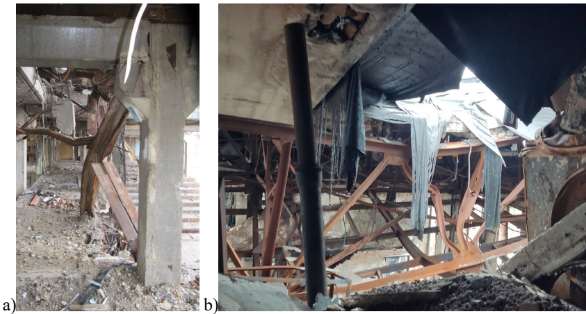
Figure 2.9 – Damage to metal structures of a multi-storey frame building: a) bending from the plane of vertical cross-ties; b) loss of cross-sectional shape and design position of the metal truss
