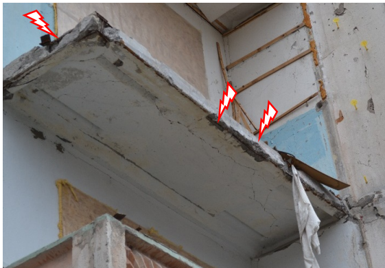
Figure 4.10 – Cracking and excessive deflection of the balcony slab of the apartment on the 3rd floor, where the explosion occurred
