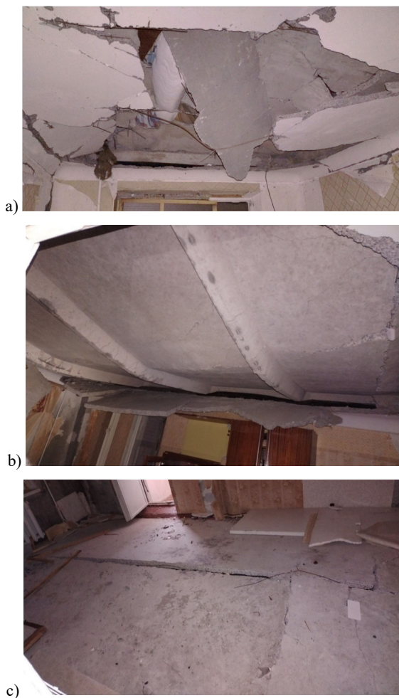
Figure 4.11 – Complete destruction of interfloor ceilings below and above the apartment in which the explosion occurred (between the 2nd and 3rd and 3rd and 4th floors) with exposure, bulging, displacement, loss of adhesion to concrete, reaching the yield point and rupture of reinforcing bars
