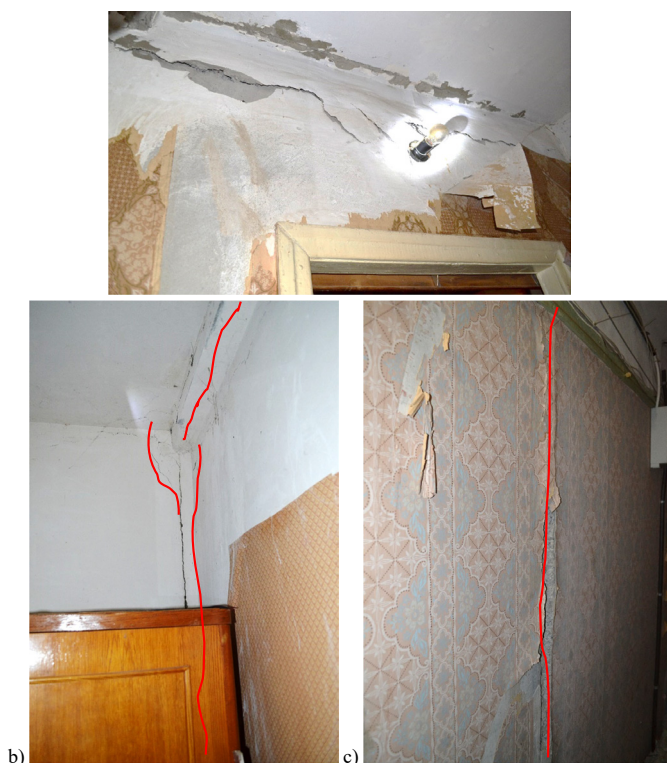
Figure 4.6 (a-c) – Formation of through and surface cracks, fragmentation, peeling of reinforced concrete structures and destruction of the filling of the joints between them within the 1st and 5th floors in the rooms above and below the apartment in which the explosion occurred
