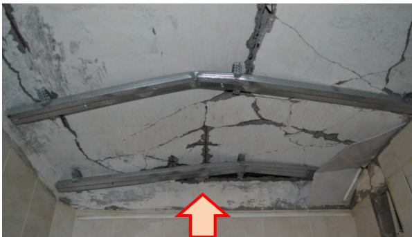
Figure 4.13 – Destruction of the bathroom floor slab above the apartment where the explosion occurred
