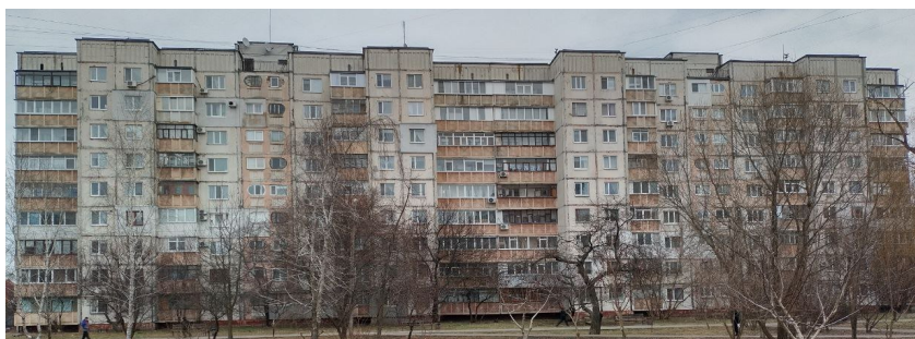
Figure 4.3 – General view of a residential building made of volumetric blocks
