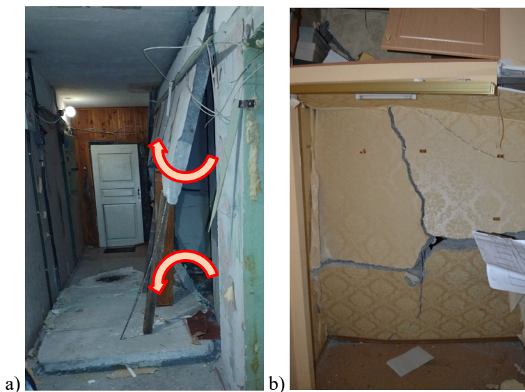
Figure 4.7 (a-b) – Destruction of 100 mm thick reinforced concrete partitions between apartments on the 3rd floor around the apartment where the explosion occurred
