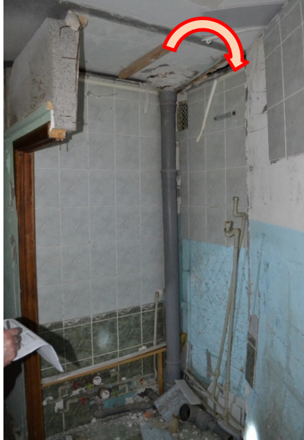
Figure 4.12 – Exit from the design position of the internal partition of the bathroom of the apartment on the 3rd floor, where the explosion occurred
