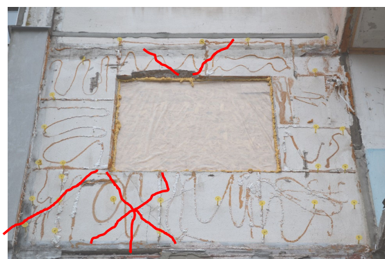
Figure 4.8 – Cracks in the body of the 320 mm thick reinforced concrete exterior wall panels on the 3rd floor around the apartment where the explosion occurred
