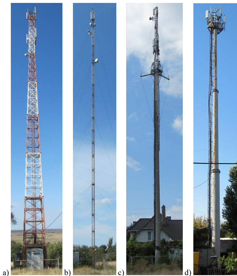
Figure 5.2 – General view of communication antenna structures: a) tower; b) mast; c) combined support; d) tubular tower
