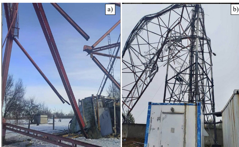
Figure 5.9 – General collapse of communication antenna structures as a result of air bombs hitting the load-bearing elements of their lower part: a) destruction of elements of the lower section of the tower; b) destruction of one post and adjacent braces
