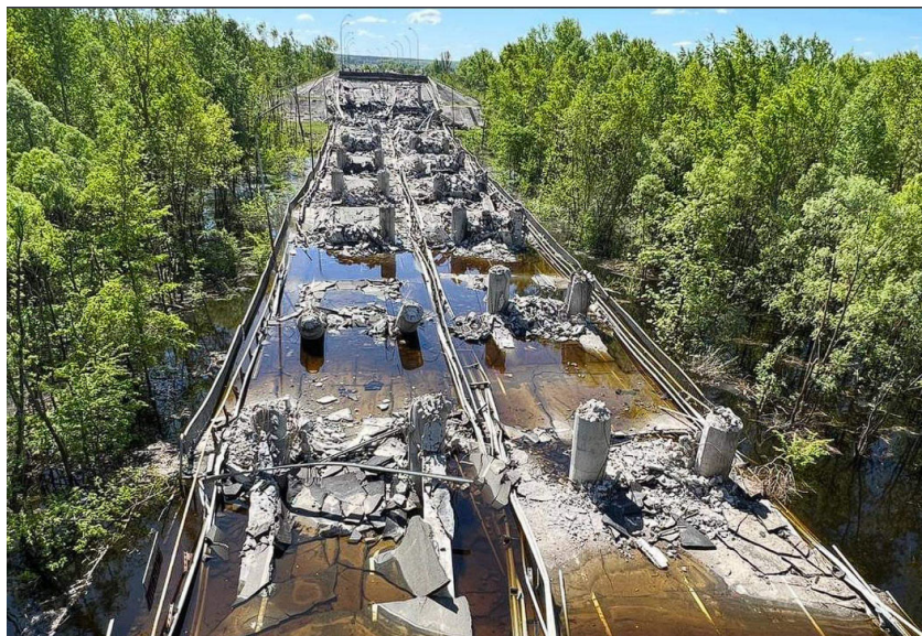
Figure 6.1 – Two large transport bridges over the Desna River were destroyed by the explosion of several large aerial bombs [57]
