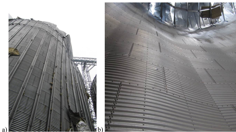
Figure 7.5 (a-b) – Loss of design position (appearance of roundness) of the wall of the cylindrical part of the silo structure No. 8 by up to 200 mm (external and internal view)
