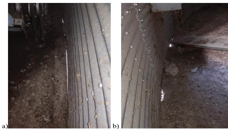
Figure 7.8 (a-b) – Formation of cracks and through holes at floor level due to displacement and movement of silo body No. 11 and local destruction of the concrete floor to a depth of h=10...50 mm
