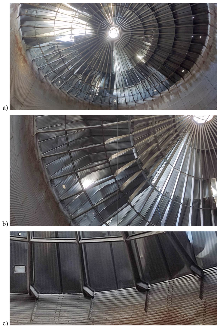
Figure 7.9 (a-c) – Destruction of the covering and purlins of the roof supporting system of the silo building No. 9 and the formation of numerous openings and cracks
