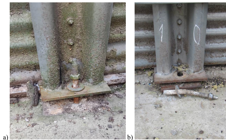
Figure 7.6 (a-b) – Separation of anchor bolts (studs) along the perimeter of the lower belt of the structure's cylindrical part, which occurred because of deformations and movements of the silo body
