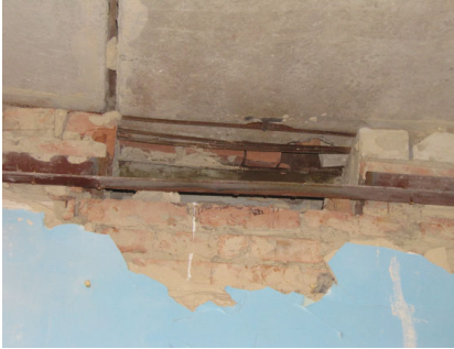
Figure 1.8 – Defect of the jumper above the slot and stress concentration
