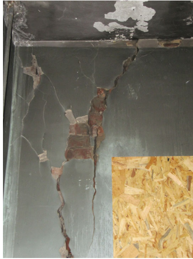
Figure 1.7 – Diagonal cracks in the section near the window opening
