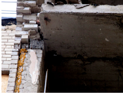
Figure 1.9 – Violation of the “wall-floor” connection and edge delaminations
