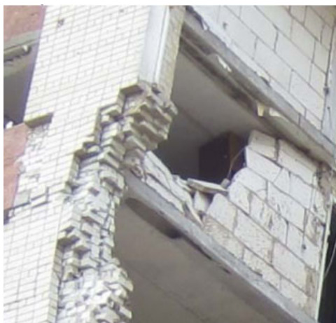
Figure 1.5 – Local wall penetration with the formation of a rectangular opening
