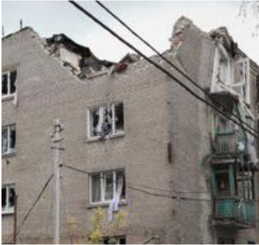
Figure 1.4 – General view of large-scale destruction of a building with a wall structural scheme after a direct hit [20]
