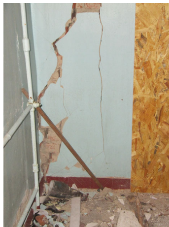
Figure 1.6 – Separation at the contact point between the block and the mortar
